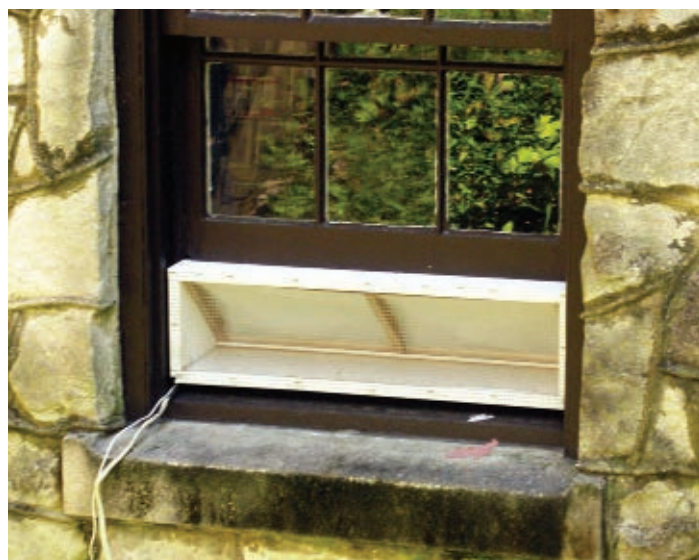
■ FIGURE 5: Outside view of a vent box.
